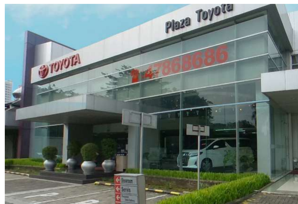
Assessment, Testing, Analisis Gedung Plaza Toyota JAKARTA
