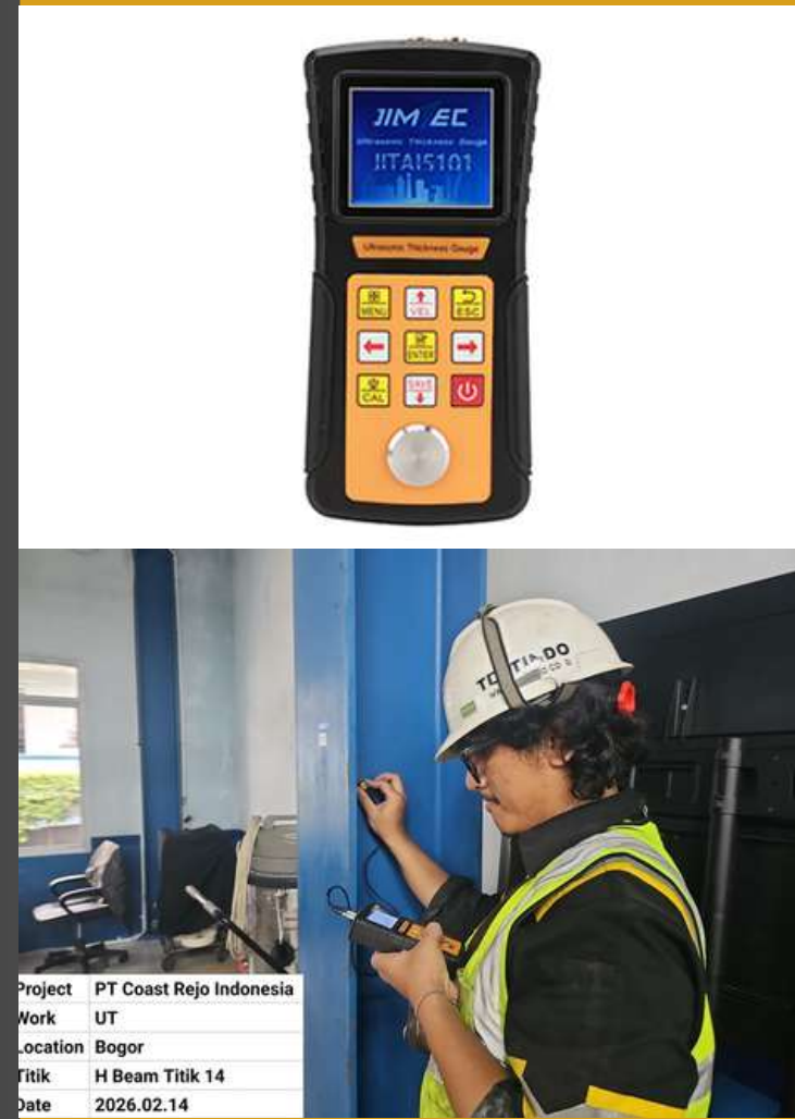
Ultrasonic Thickness Test
