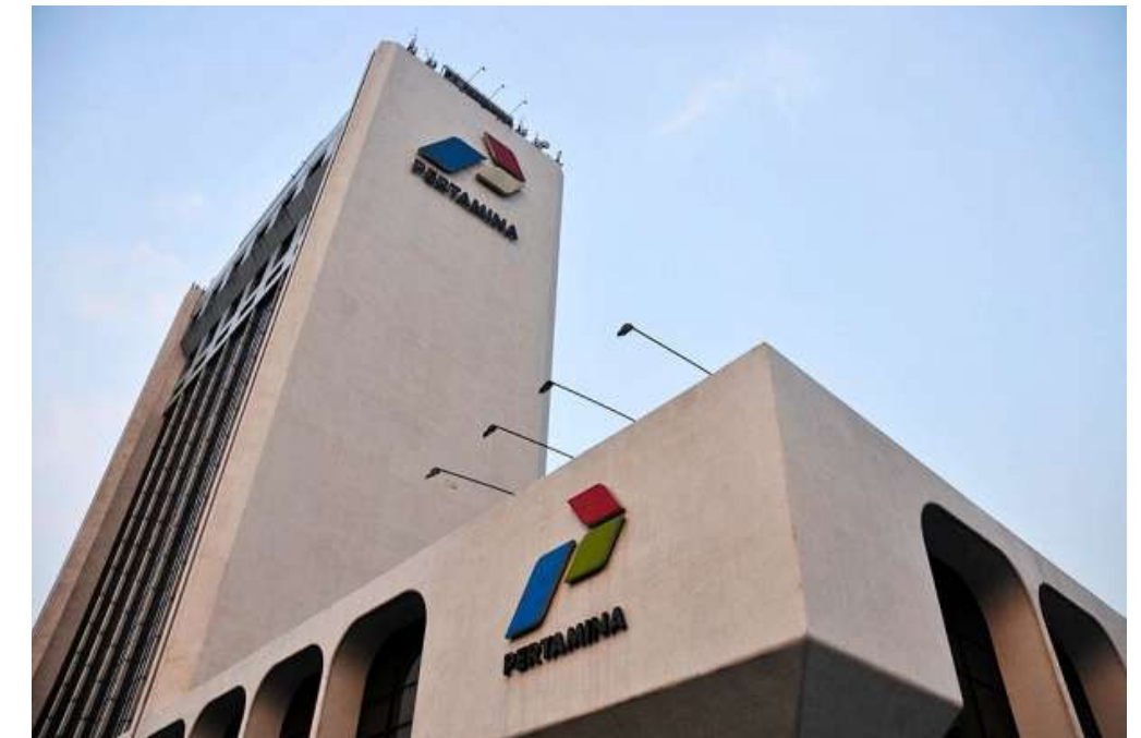
Assessment, Testing, Analisis Struktur Tower Pertamina Gambir JAKARTA
