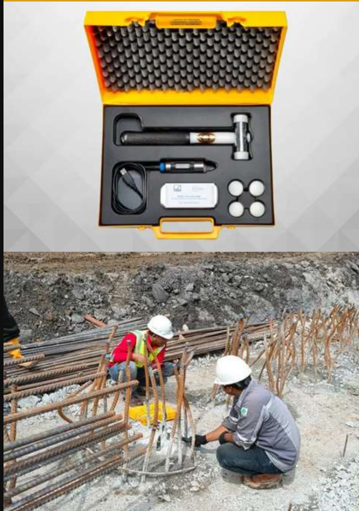
Pile Integrity Test
