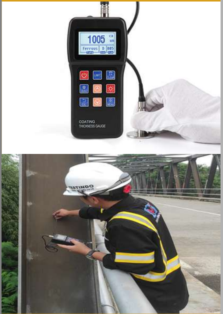
Coating Thickness Test
