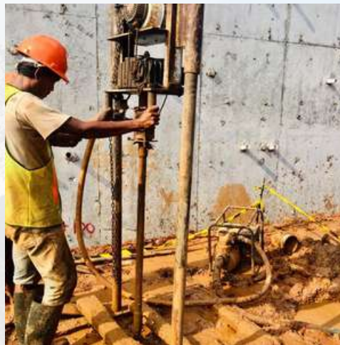
Project Instalasi & Monitoring Inclinomater - Tol Serpong Balaraja
