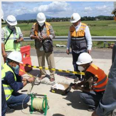
Project Instalasi & Monitoring Inclinomater - Tol Serang Panimbang
