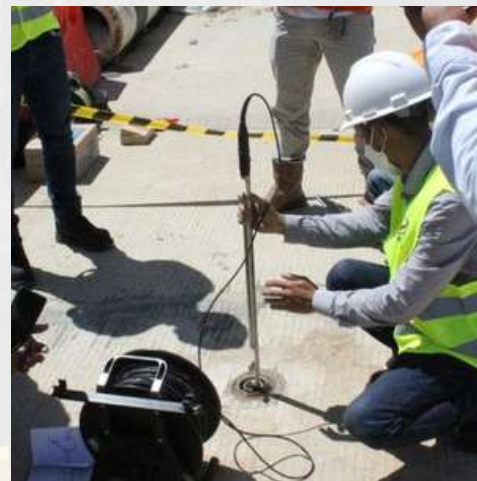
Project Instalasi & Monitoring Inclinomater - Tol Serang Panimbang
