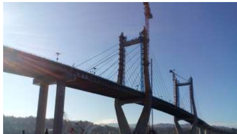
Online Monitoring Jembatan Merah-Putih (Structural Health Monitoring System/SHMS), Ambon – Maluku, 2016
