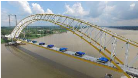
Online Monitoring Jembatan Kukar (Structural Health Monitoring System/SHMS), Tenggarong – Kalimantan Timur, 2015
