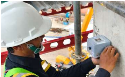
Structural Health Monitoring System (SHMS) Jembatan Tol Sedyatmo - PT PP Persero Tbk
