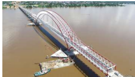
Online Monitoring Jembatan Tayan (Structural Health Monitoring System/SHMS), Pontianak – Kalimantan Barat, 2015
