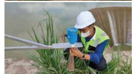
Application Radar Water Level Sensor on dam
