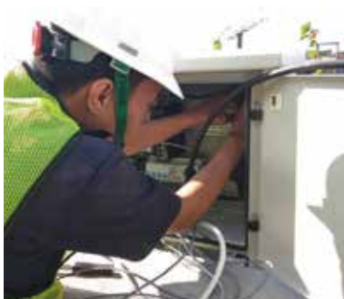
Structural Health Monitoring System Jembatan Tol Ir Wiyoto Wiyono
