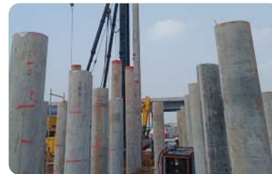
Pile Vibration Monitoring
