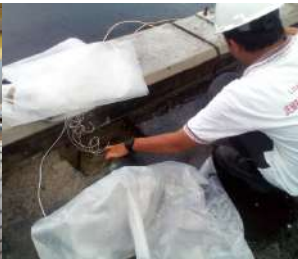
Installation of Sensor at Merah Putih Bridge
