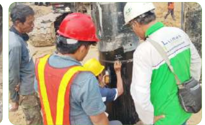
NDT Project for Welding Joints of Pilings
