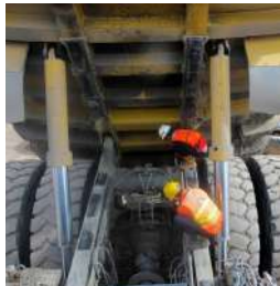
Installation of Analyzer Instrument at PT Pama Persada
