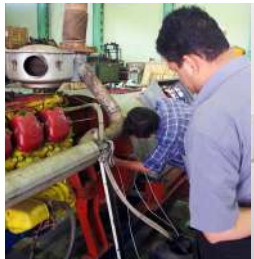
Installation of Monitoring Systems Instrument at PLN Pusharlis
