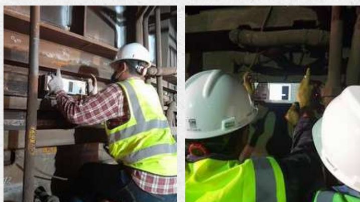
Project Ultrasonic Concrete Tomography (UCT) at Furnace 3 UBPN Southeast Sulawesi
