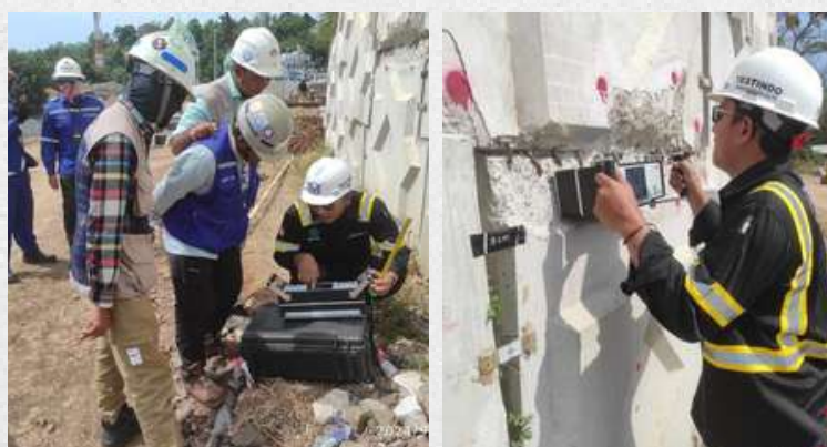
Project Ultrasonic Concrete Test, Repair of GSW Steam Power Plant in Suralaya, Cilegon
